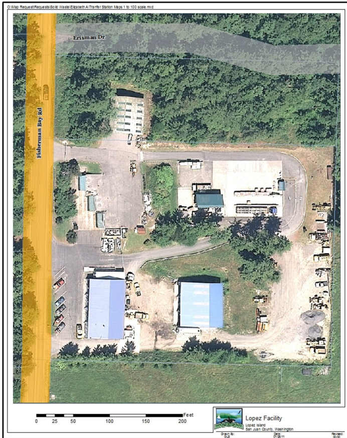
Figure 6.3 Lopez drop-box facility
